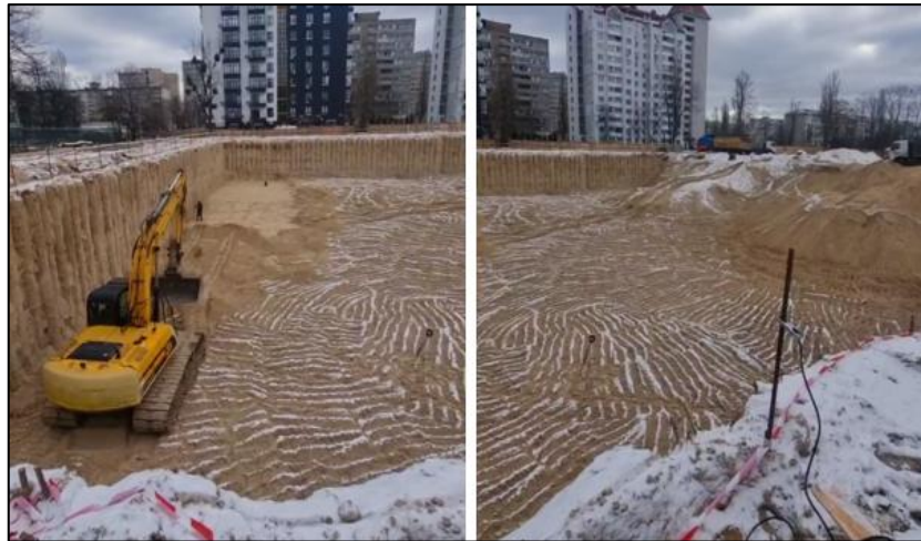
Fig. 2. Process of excavation development
